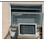
**Through-the-window air conditioners** (also: compact or through-the-wall AC) are widespread in the USA, but of no importance in Europe. They are too compact to be efficient and need an opening in the insulation.
